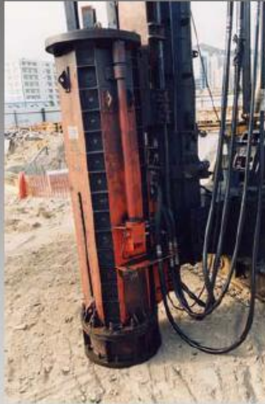
Hydraulic hammer for driving pile
