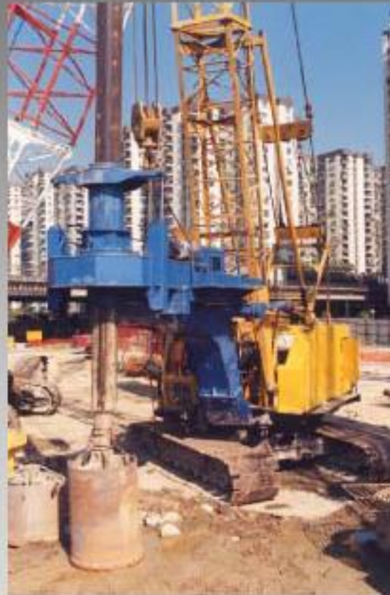
Medium dia. pile formed using bucket barrel
