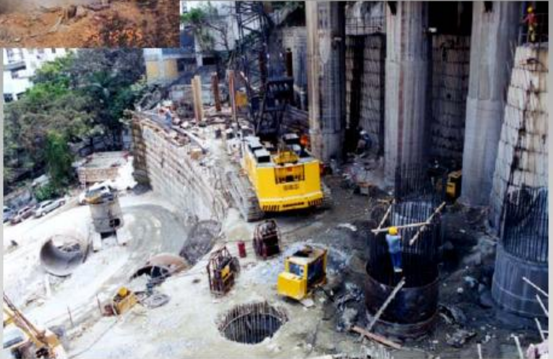
Hand-dug caisson working in sloped site
