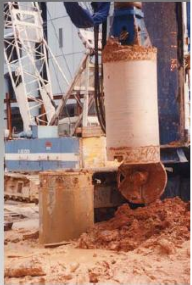
Bucket barrel taking soil from the borehole
