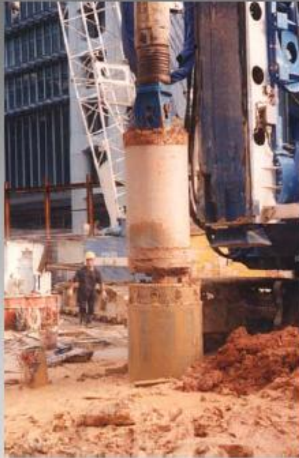
Bucket barrel taking soil from the borehole
