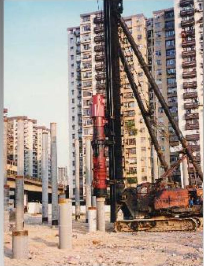
Precast circular-section pile driven by diesel hammer
