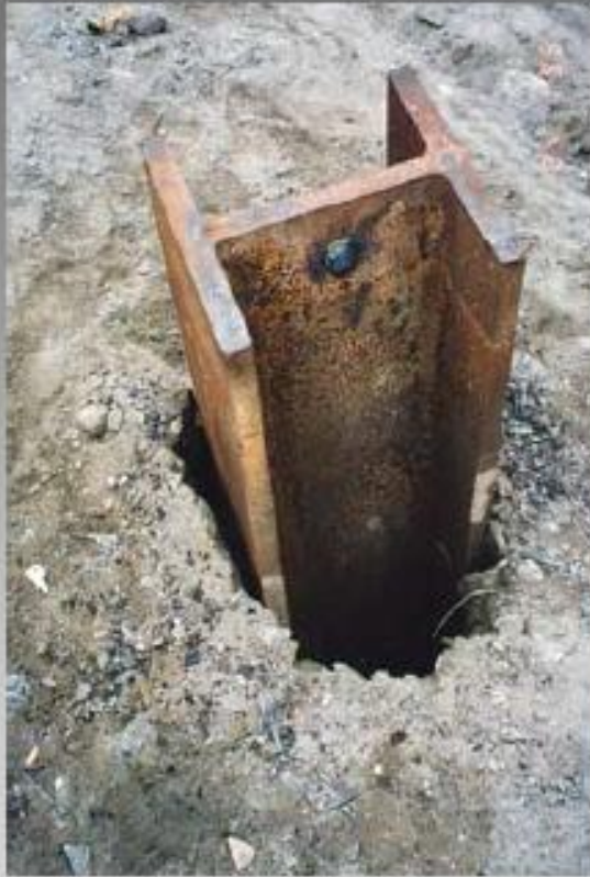
Inserting H-pile after pre-boring
