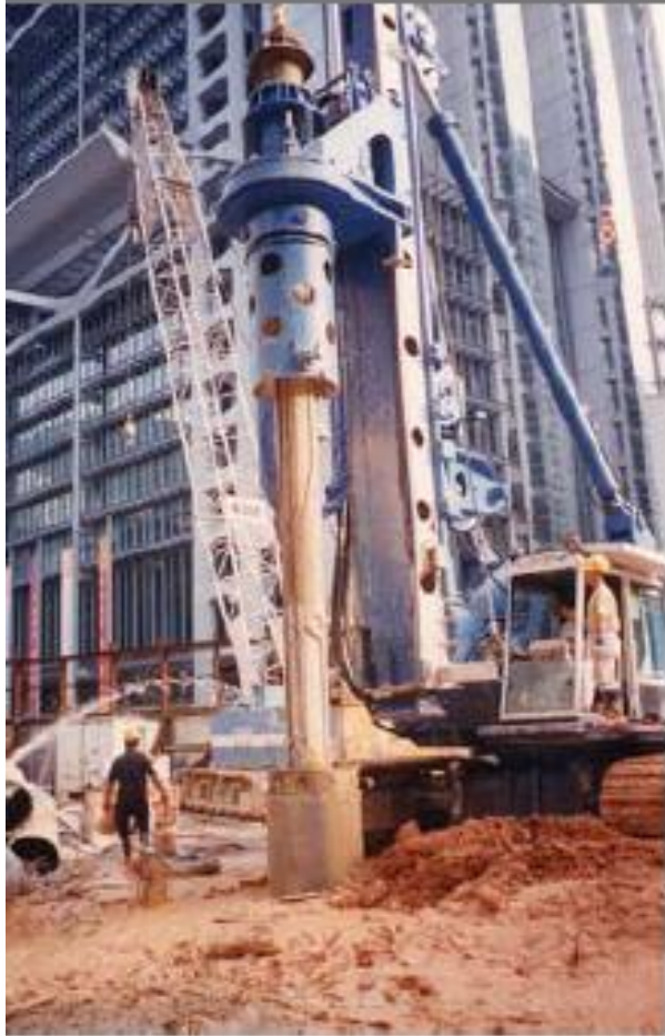
Bucket barrel taking soil from the borehole
