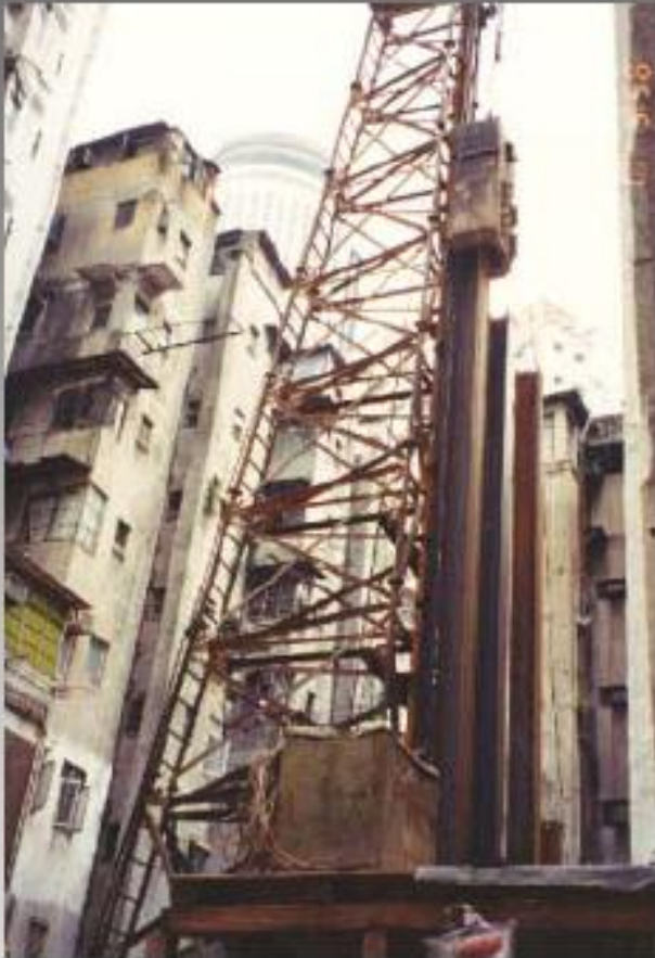
H-pile driven using gravity drop hammer
