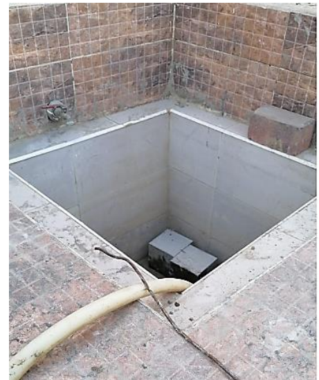
Water Curing Basin (2)
