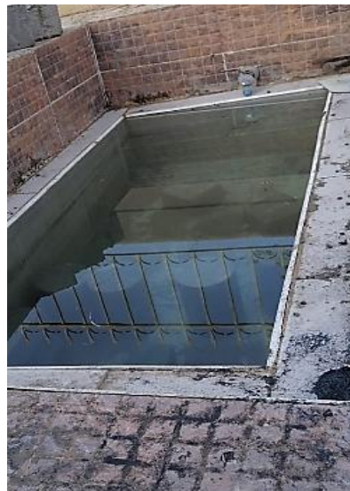
Water Curing Basin (1)
